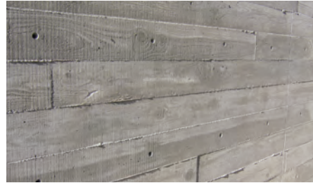
Figure 39 Example of concrete finish
