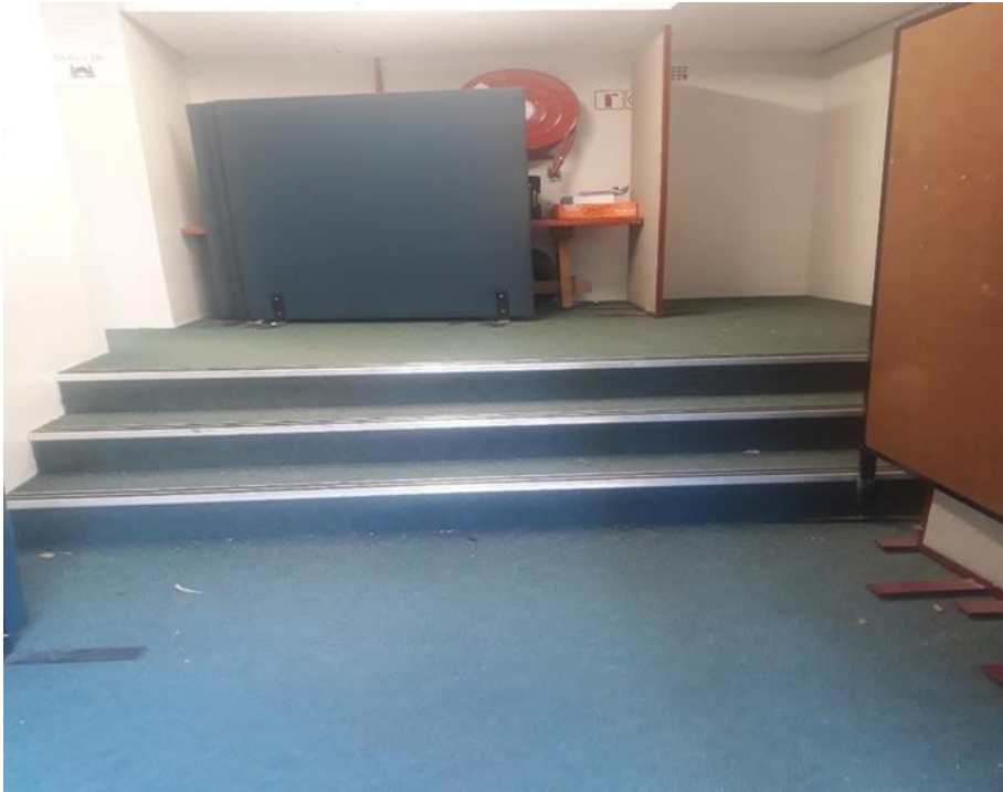
Figure H. 3: Second entrance into the University of Cape Town prayer facility
