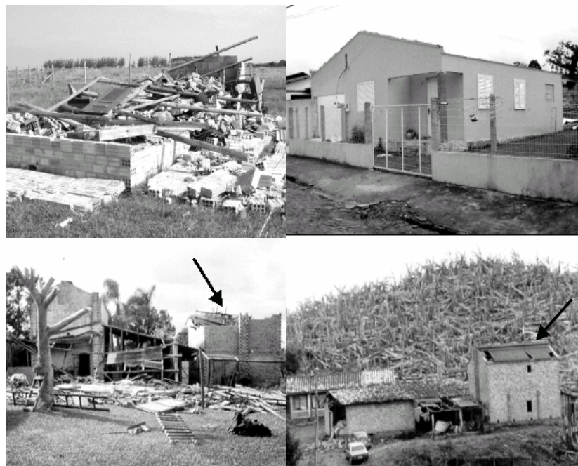
Figure 1.6: Examples of damage caused by Hurricane Catarina (Marcelino et al. , 2004: 5)
