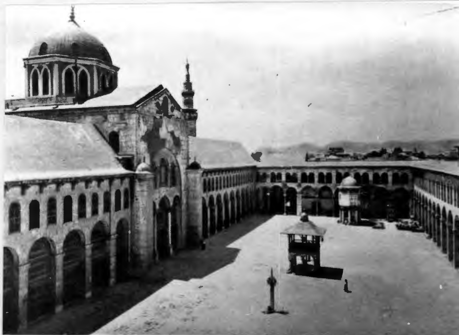
DAMASCUS: the Great Mosque. interior looking west
