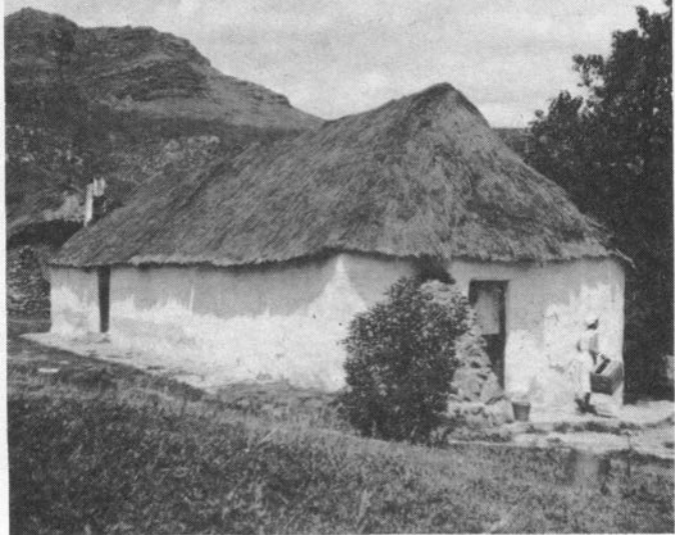
Fig 14: Eselshoek. A dwelling with gable entrance and a kitchen entrance at the opposite end. Built after Poortermans made his painting but typical of many Piquetberg houses which he illustrated.
