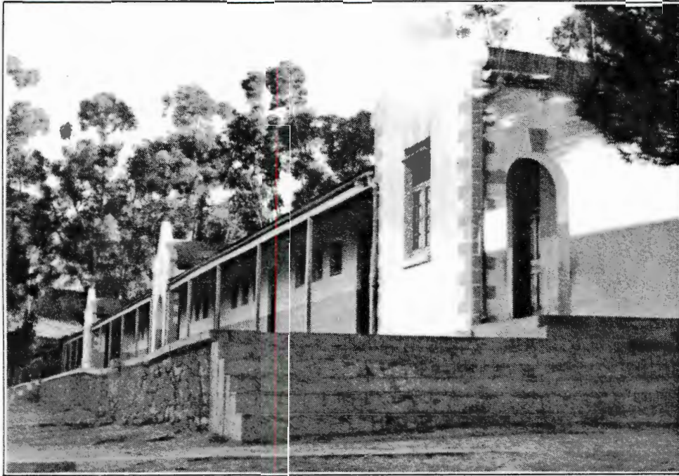
Figure 24 The three gabled school
