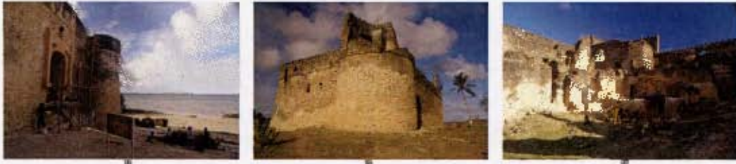
Figure 5.1: The Gereza: East façade (a), South and West façade (b), inside court (c)
