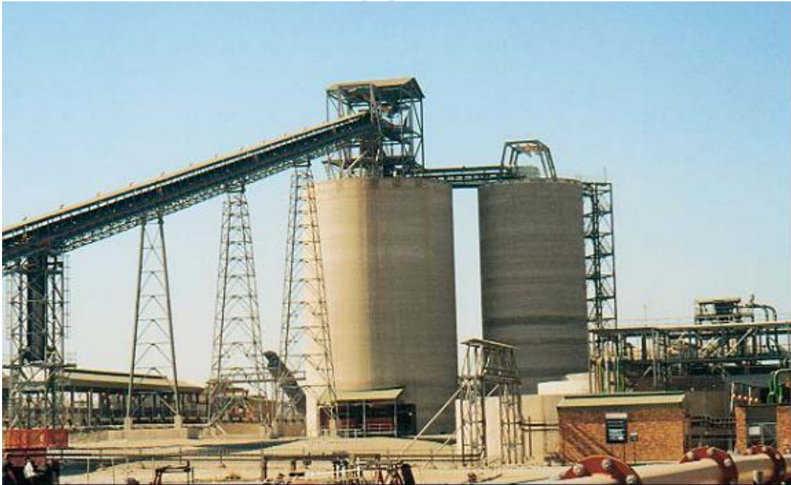
Figure 1.4 Coarse ore and fine ore silos at the Waterval UG2 concentrator (Davies, 2002).
