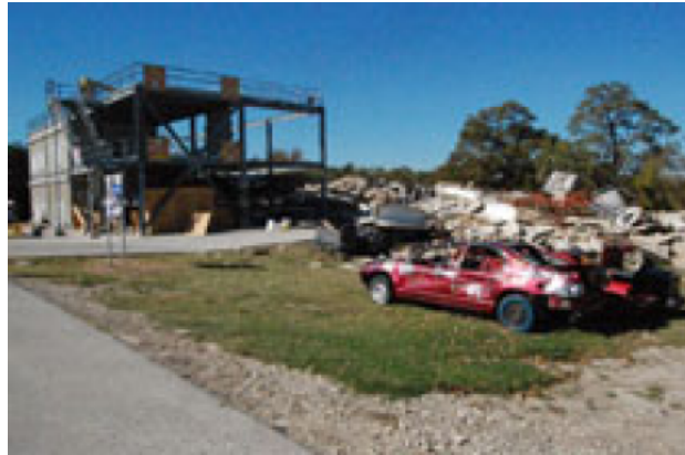
(a) Unstructured image of collapsed car parking lot
