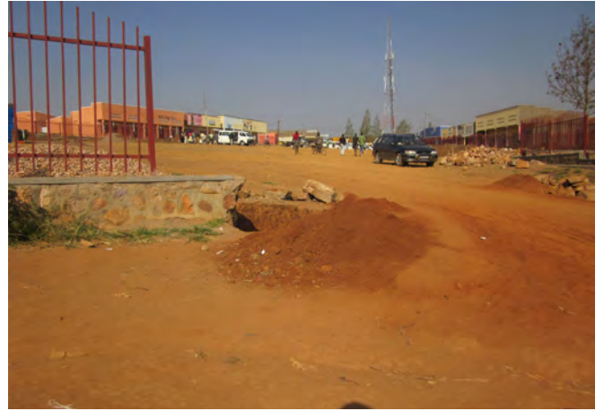
Photo 5.2: The new taxi park (Source: the author)
