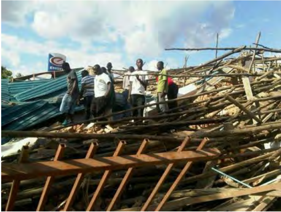
Photo 5.9: Collapsed building (Source: Ndaka 2013)
