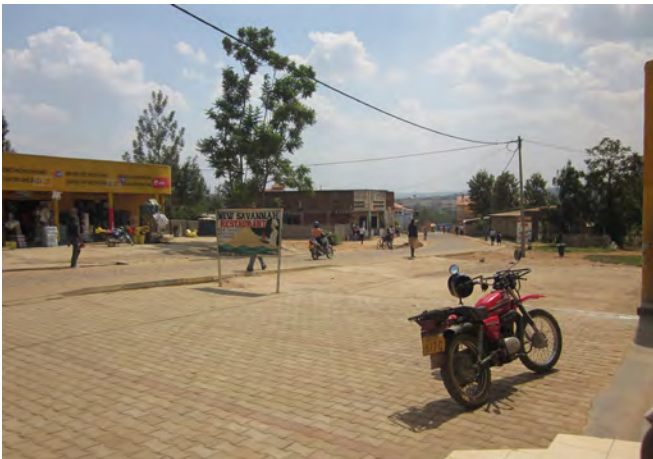
Photo 5.3: A recently-paved road (Source: the author)
