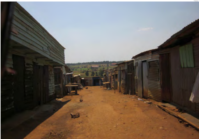
Photo 5.5: The temporary market (Source: the author)
